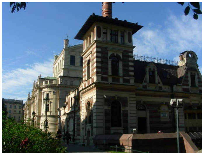
Fig. 4. The power station of the Municipal Theatre. Fot. J.Kukulak
