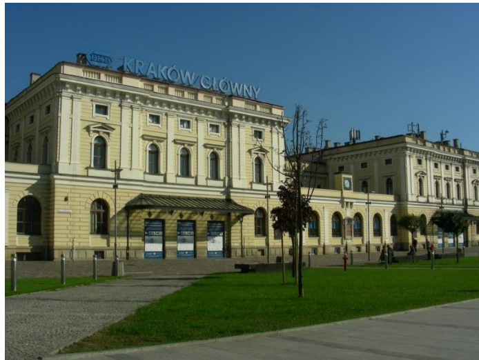
Fig. 2. Main building of Train Station in Cracow. Fot. J.Kukulak
