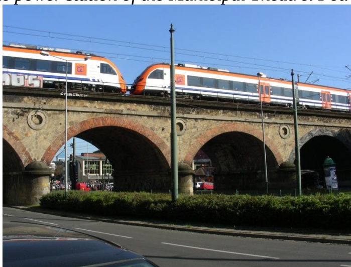
Fig. 5. Viaduct over the Grzegórzecka street - the old railway bridge over the Vistula River. Fot. J.Kukulak
