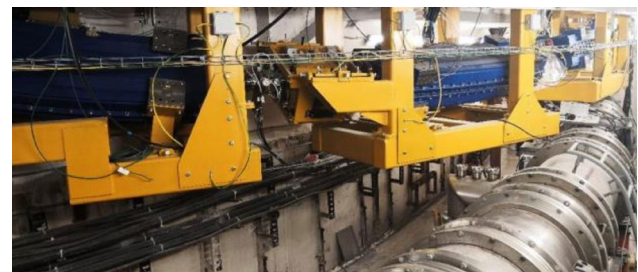
Figure 15: The Booster-Nuclotron transfer line.
