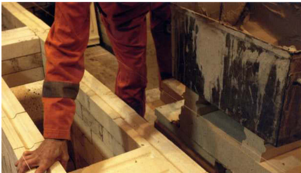
Fig. 1. Lining of a partition wall of anode furnace with BorABF products.
