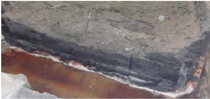
Fig. 4. Delamination of cathode blocks in 3 year old cell causing failure due to high iron
