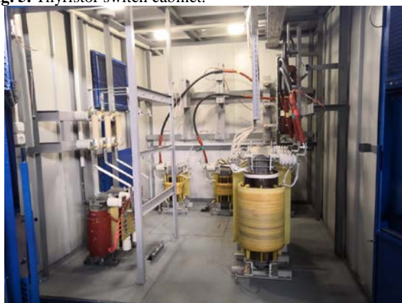
Fig. 6. Power transformer compartment.
