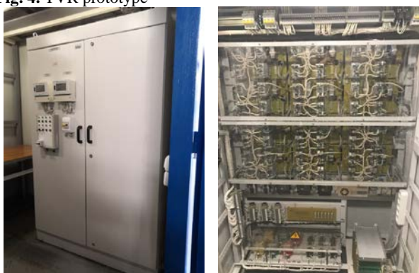
Fig. 5. Thyristor switch cabinet.
