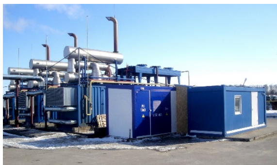
Fig. 1. Experimental power system for testing the combined work of ESS-10-1200-400 and GEG.
